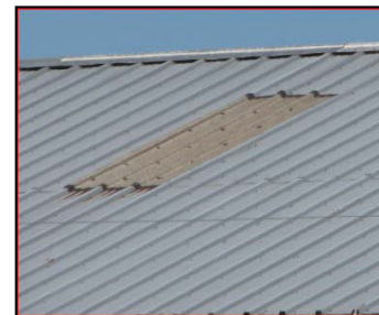
Skylight panel in a metal roof.
