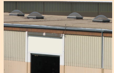
This is an example of skylights on a flat commercial roof.
