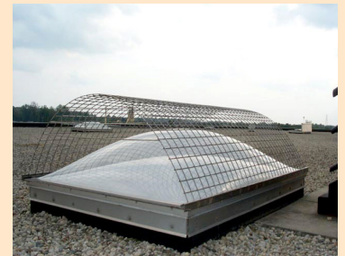
This is an example of a skylight with a safety cover.
