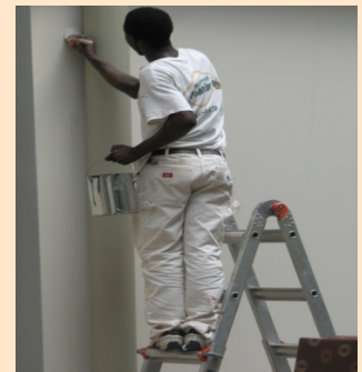
Unsafe: Keep three points of contact with the ladder.
