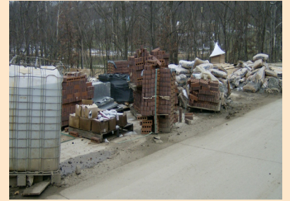
Establish a supply staging area and keep it organized.
